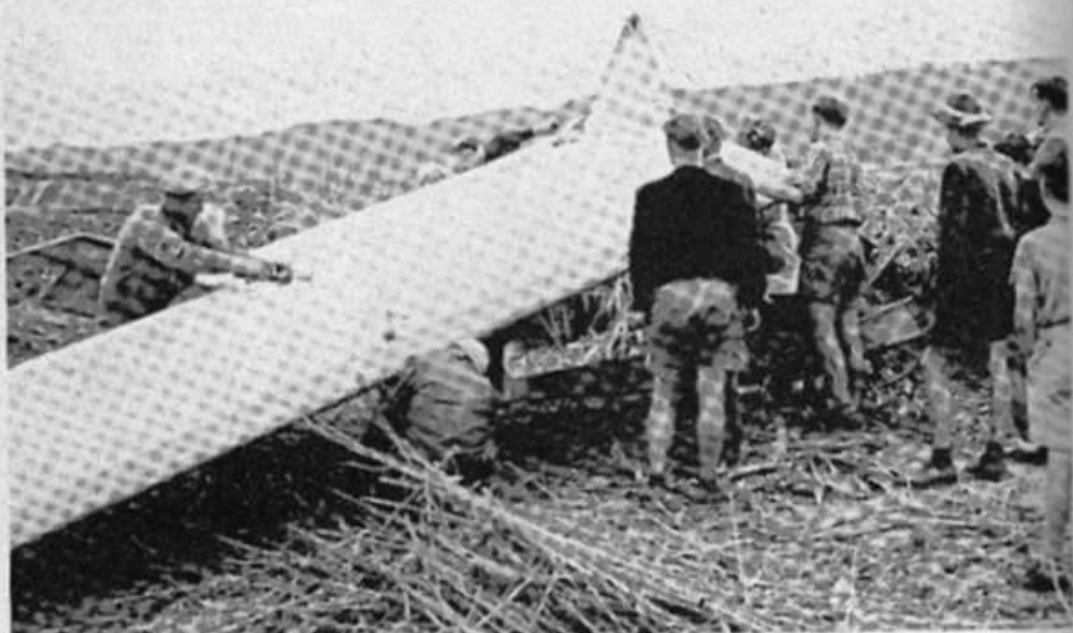
SG-Bruch in Heiningen
